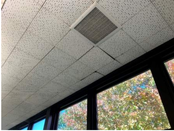
Photo A20 – Asbestos Ceiling Tile
