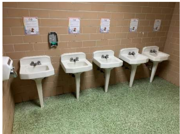
Photo A07 – Typical Restroom
