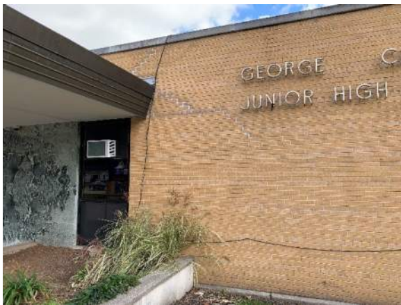
Photo A12 – Tuckpointing at West Elevation
