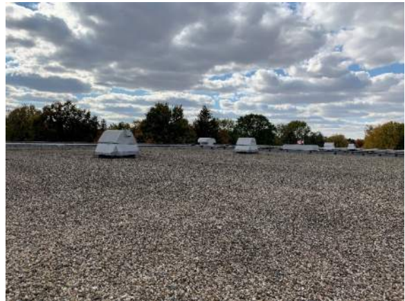
Photo A17 – Gymnasium Roof (Upper)
