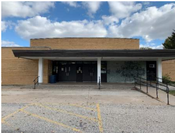
Photo A_C – Main Entry (Exterior)
