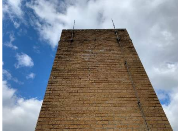
Photo A15 – Masonry Repair, Chimney
