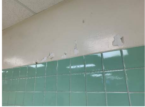
Photo A21 – Painted Finish (at Corridor)
