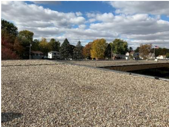
Photo A16 – New/Old Roof (Lower)
