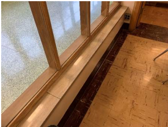
Photo A18 – Terrazzo & Asbestos Floor Tile
