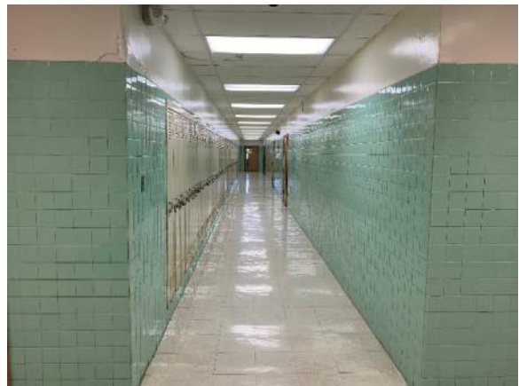
Photo A05 – Dead End Corridor
