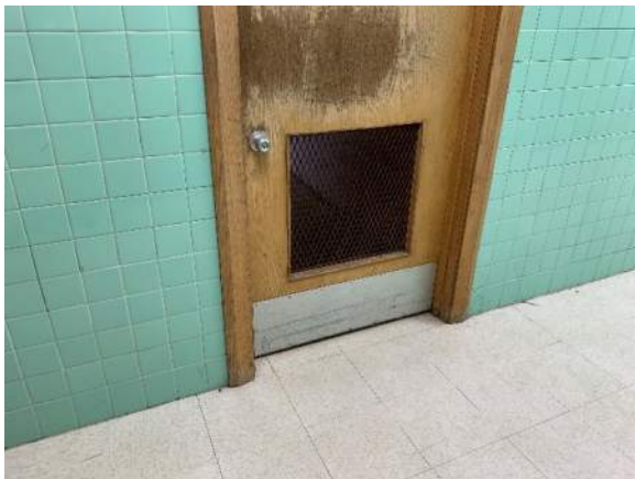
Photo A04 – Corridor Door w/ Grill
