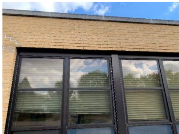
Photo A13 – Tuckpointing, Typical
