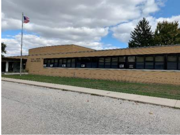
Photo A02 – West Elevation
