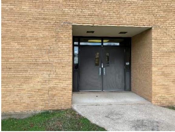
Photo A14 – Masonry Repair, East Elevation
